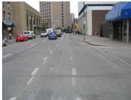
Bike lane ends and sharrow begins on the right
